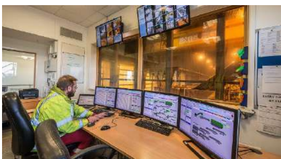
(1) CONTROL SYSTEM AUTOMATIC 24/7
