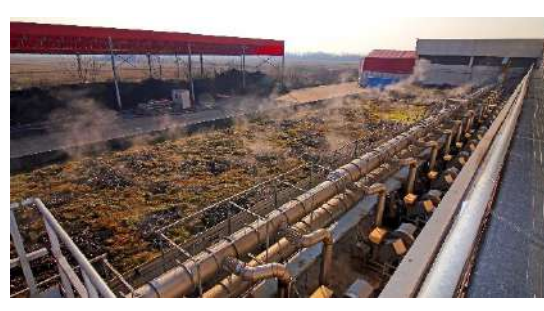
(3) BIOFILTER FOR PROCESS AIR TREATMENT
